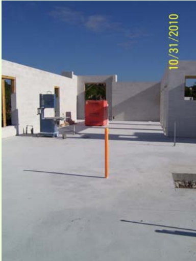
What's that orange pipe sticking up?
